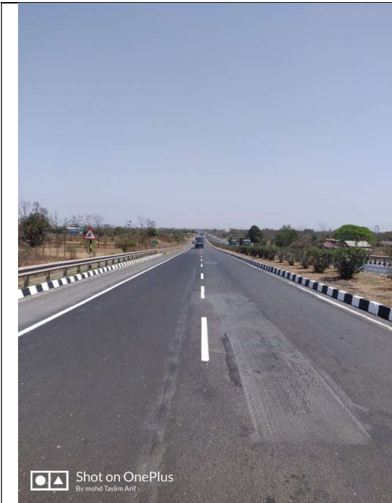
BC work after milling were completed also the road marking
